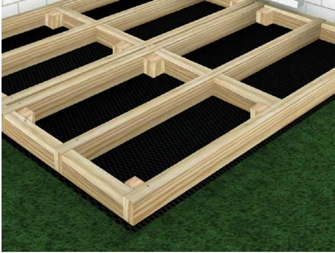
**1** We recommend leaving a space of **450-500mm between rows of Joists**. Deck Tape can be applied and to protect Timber Joists from moisture at cut the ends. For raised Decking areas, ensure Posts are placed at 1m intervals across the installation for adequate support.
