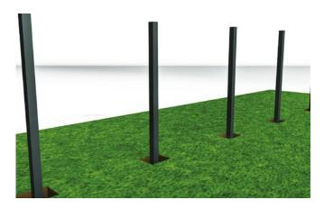
Prepare your area by removing any stones, debris or hazardous material. Dig the Fence Post holes to 25% of the Post height. The Fence Posts must be a maximum of 1.8m apart to ensure they can support the Fence Panels. Run a piece of string from the first Post to last Post to make sure they are positioned square to each other.
