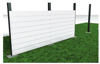
**Z** As you start to add more Panels ensure each Panel is 100% level before fixing. Each Fence Panel slots on top of the Panel previously fitted. (Example shows 3.6m Fence Panels with Fence Post in between).
