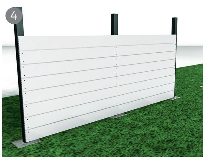
4 As you start to add more boards ensure each fence panel is 100% level before fixing. Each fence panel slots on top of the board previously fitted. (Example shows 4m fence panels with fence post in between).
