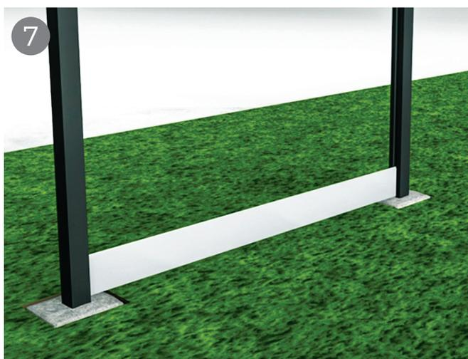
When using the cut method the fence panels need to be cut into 2 metre lengths. The posts must be no further apart than 2 metres.
