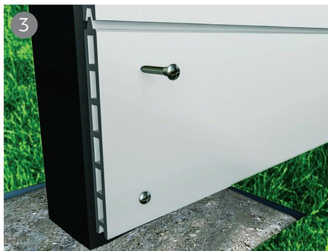
3 When adding the first fence panel board, ensure it is 100% level before fixing to posts. Screw the top and bottom of each fence panel to the fence posts behind.
