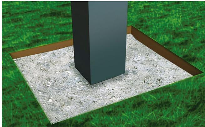
**3** Make sure every Fence Post is 100% level before using postcrete. Fence Posts must have at least 25% of their height concreted into place.
