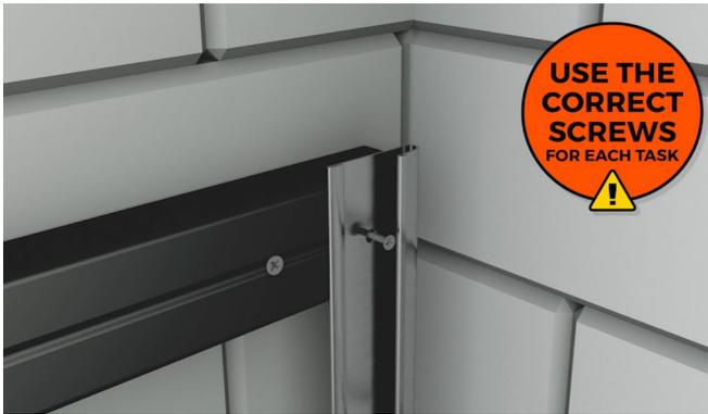
**4** Attach a Starter Strip to the right side of each Batten, as this will give the first Cladding Board something to sit on. You may wish to pre-drill a pilot hole into the Composite Batten and attach the Starter Strip using a screw that is at least 15mm long. Ensure that each Strip is level with the next and that the first Board sits level on the Strips before continuing to the next step.
