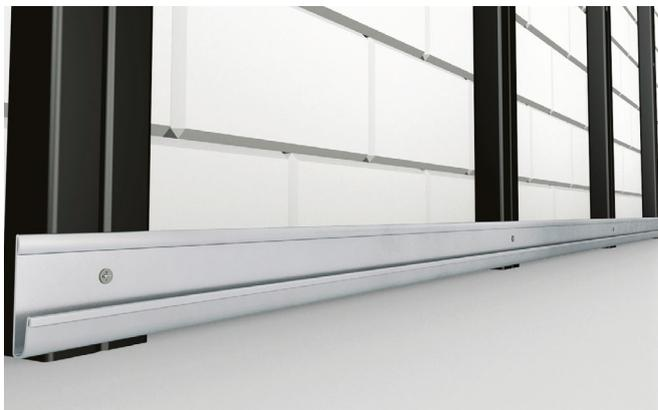
**3** Attach a Starter Strip to the bottom of each Batten. This will give the first Cladding Board something to sit on. You will need to pre-drill a pilot hole into the Composite Batten and attach the Starter Strip using a screw that is at least 15mm long. Ensure that each Strip is level with the next and that the first Board sits level on the Strips before continuing to the next step.
