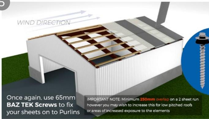
Sheets should be overlapped by the next sheet in the run by at least two profile or corrugations ('side laps'). Adjacent runs of sheets should overlap each other by at least 250mm ('end laps'). Please note, we can only supply a maximum of 6 metres. If you require a longer length, its recommended to do a two sheet run.
