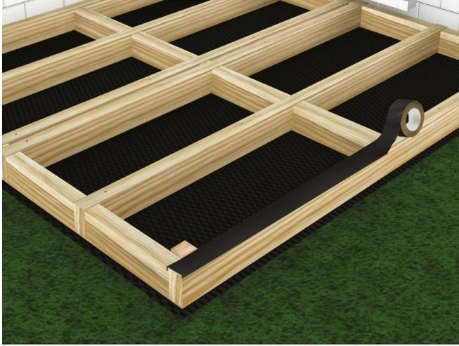
**1** We recommend leaving a space of **45-50cm between rows of Joists**. Deck Tape can be applied and to protect Timber Joists from moisture, cut the ends.
