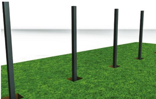
**2** Prepare your area by removing any stones, debris or hazardous material. Dig the Fence Post holes to 25% of the Post height. The Fence Posts must be a maximum of 1.8m apart to ensure they can support the Fence Panels. Run a piece of string from the first Post to last Post to make sure they are positioned square to each other.
