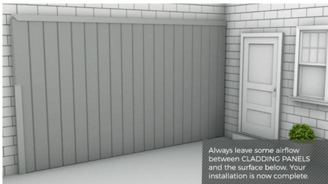
**8** Depending on your installation, you may want to finish off the edges using Trims to give you a lasting professional look. There are a range of Trims available in all colours to complement your Cladding Boards, which can be secured to your installation by glue.
