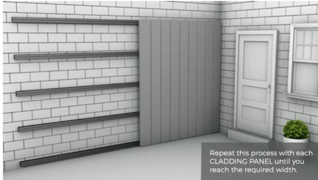
**7** It is possible to fit your Boards side by side by simply butting the two ends up together. You may need to install more Battens if you wish to do this, as each Board will need to be supported on a Batten where it meets the next Board. Continue to fit the Cladding Boards in this manner until you have completely covered the area you want.
