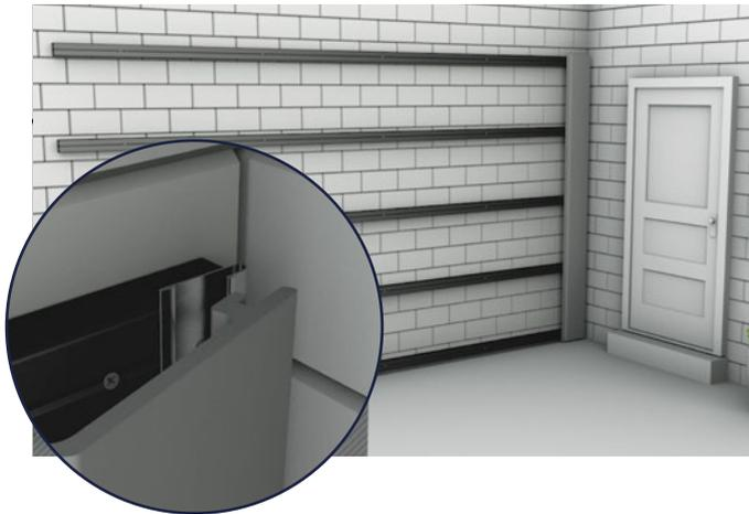
**5** Place the first Wall Cladding Board on to the Starter Strips. Mark and then pre-drill pilot holes through the fixing groove of the Board into the Composite Batten below. Secure the Boards using a screw at least 30mm in length, ensuring that the Board is fastened securely on each Batten that it touches. Secure these fixings by hand, as it is important not to over-tighten the screws and risk splitting the Board.
