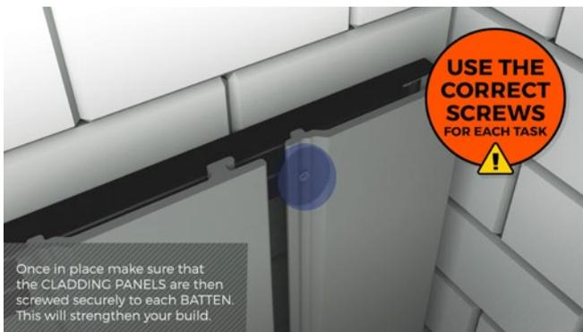
**6** Ensure that the section between the Battens remains empty allowing air to flow beneath the Boards. Slot the second Board onto the first and repeat the fixing process ensuring that the second Board is fitted securely in place on each Batten.
