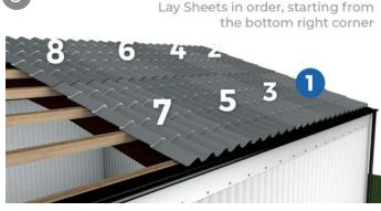
For a two-Sheet run, Sheets should be laid in a particular order starting at the eaves in the bottom right corner and then installing to the ridge. If the first Sheet is not laid perpendicular to the eaves and ridge, adjustments will have to be regularly made when laying other Sheets and a 'saw tooth' effect at the eaves will occur.
